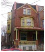
tectural details. The exterior brickwork has been repointed and steam cleaned, and a multicolored paint scheme applied to the exterior wood and metal details. The original porch balusters have been reproduced and are primed, awaiting installation in better weather." Fortunately, a break in the weather made that last touch possible before the award presentation.
